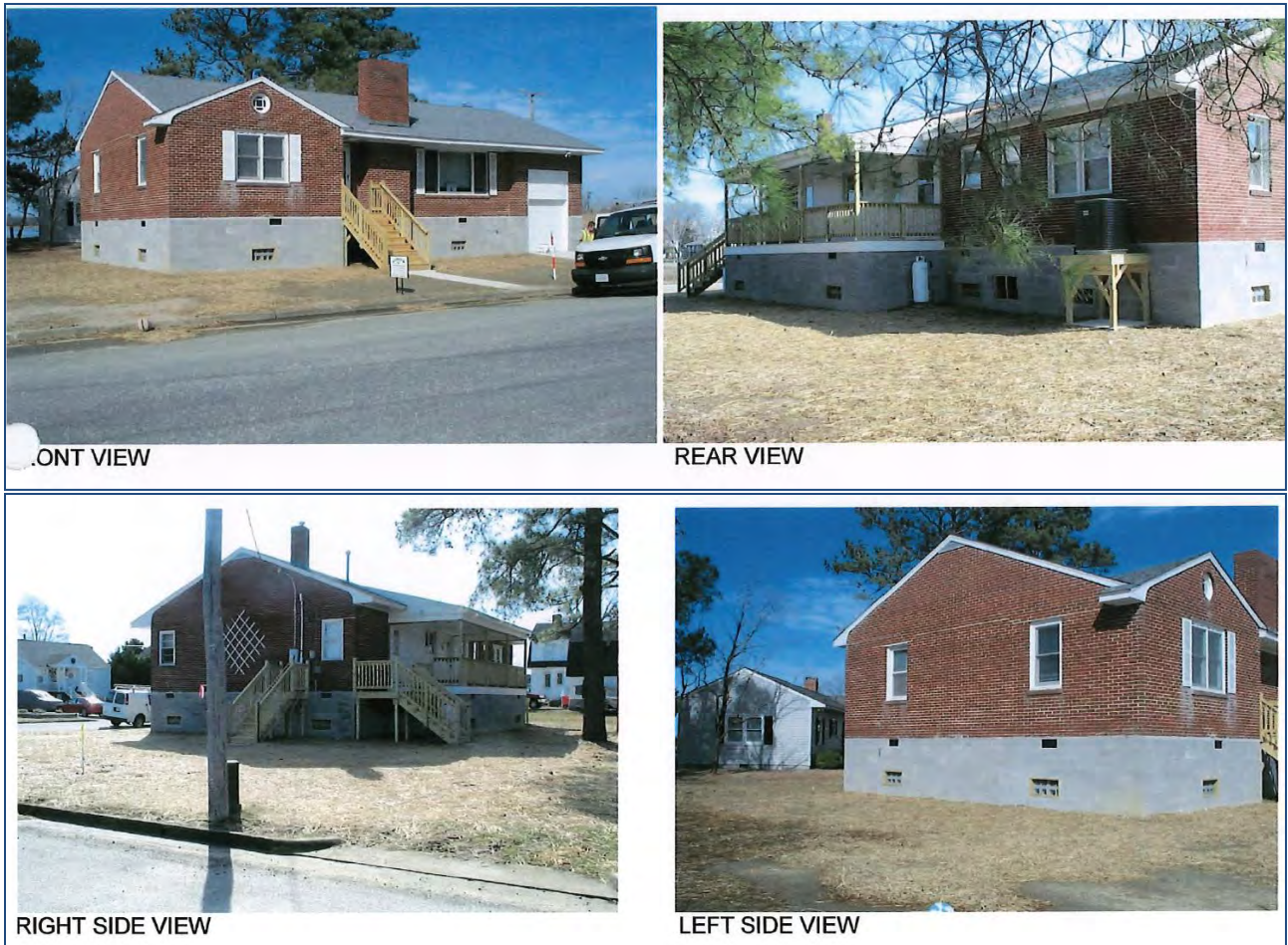
Figure 122: Photos of Kirby Street home after being elevated.
